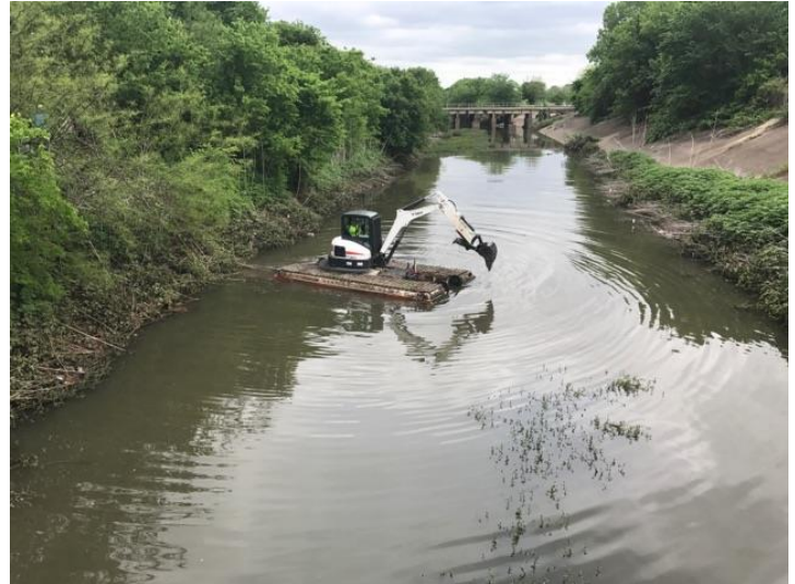
Figure 52. Example amphibious excavator (Dennis Fischer).
