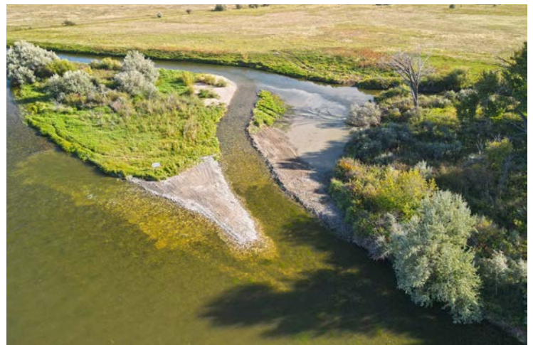
Photo 10. Above Rattlesnake Island side channel with narrowed channel & modified departure angle (post-construction, 2866 cfs).
