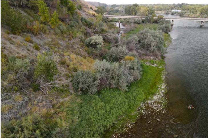
Photo 1. Saint Xavier Bridge side channel at 2865 cfs (pre-construction)
