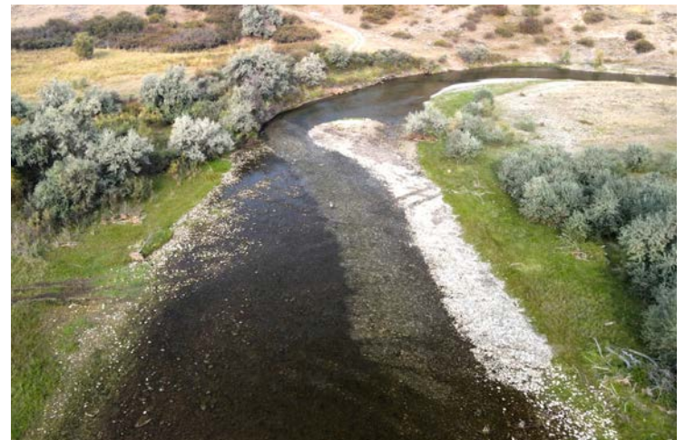
Photo 4. Narrowed and deepened riffle in Cline's channel (post-construction, 2865 cfs).
