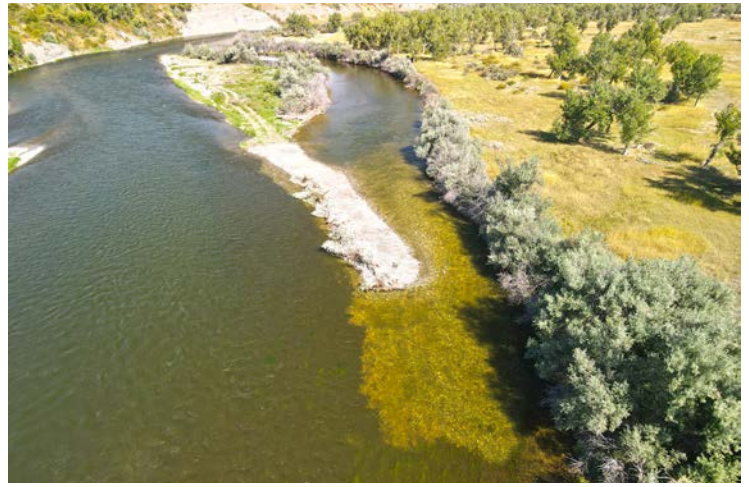
Photo 6. Narrowed entrance to “Across from Turtle Rock” side channel at 2868 cfs (post-construction).
